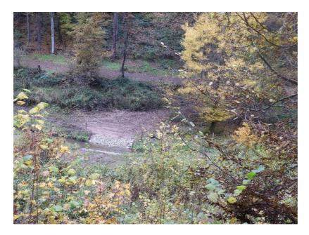
Picture 2: A ford built as part of the LIFE Biocorridors in the northern Alsace. The action aims at reducing the erosion of riverbanks and at providing crossing points in order to reduce diffused pollution along the tributaries of the River Sauer SAC
